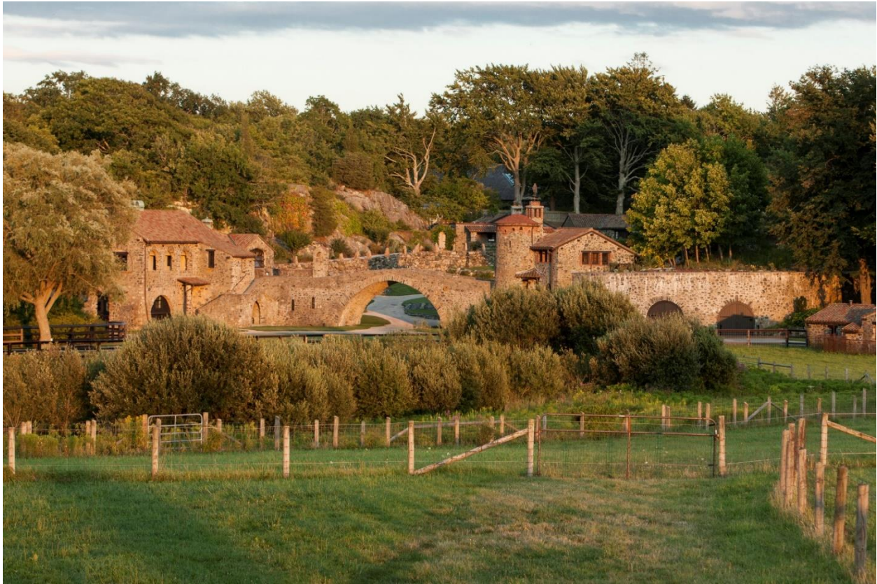
The SVF Foundation property as it looks today on Harrison Avenue in Newport. (Photo provided by SVF)
