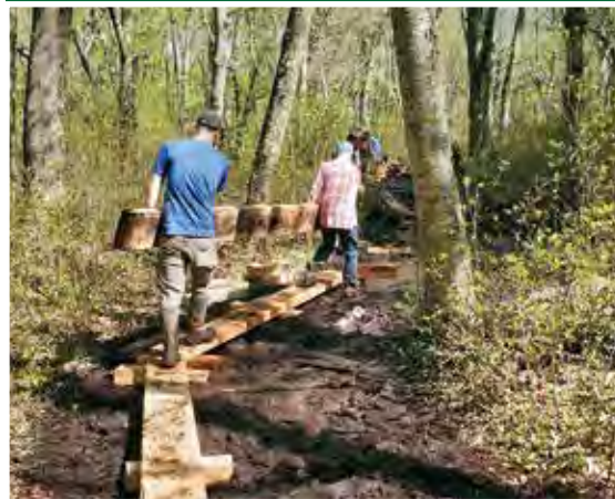
ALT staff and volunteers built 600' of new bog bridges and resurfaced 1,400' of existing trail.
