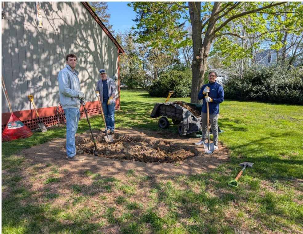
Digging out the depression. A big thank you to the volunteers who helped build the rain garden!
